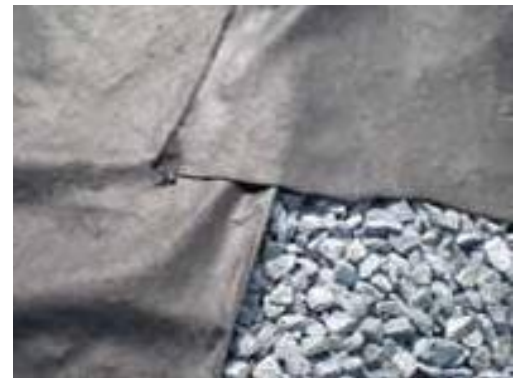
Fig 7: Overlap Geotextile by minimal 12" (300mm) or more.
