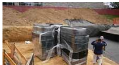
Fig. 3 Installation can be speeded up by either assembling the tanks in the excavation or placing the preassembled tanks in the excavation.
