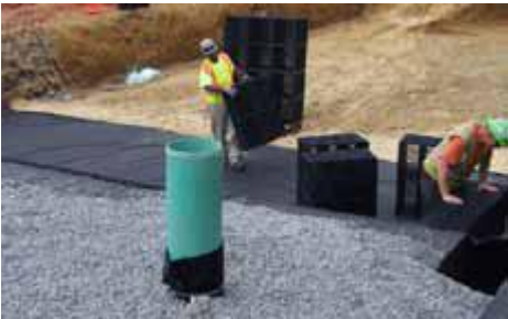
Fig 11: Installed inspection Port
