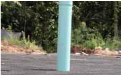
Fig. 16 Installed maintenance port
