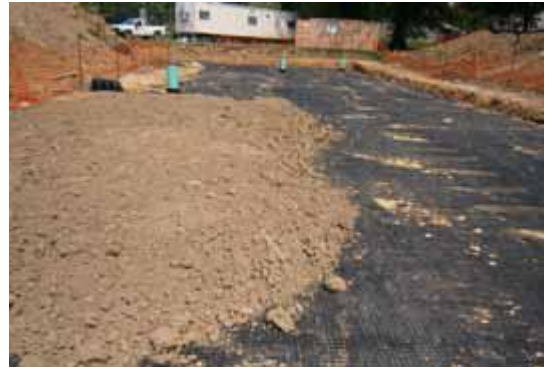
Fig. 25 Overlap Geogrid 18" or as required by plans.
