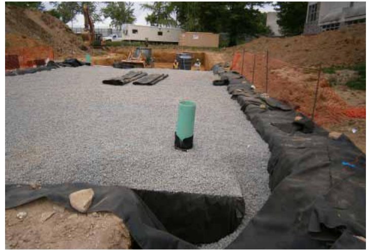
Fig. 24 Use an LGP dozer to push backfill over Ellipse Tank units.
