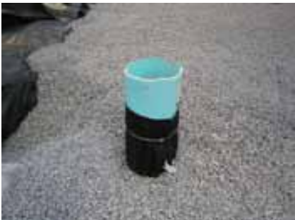
Fig. 17 Install port into R-Tank..
