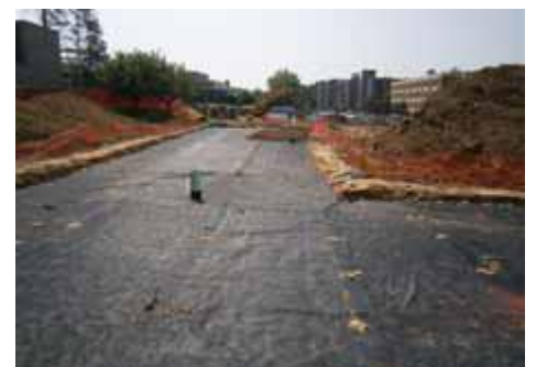
Fig. 25 Overlap Geogrid 18" (300mm) or as required by plans.
