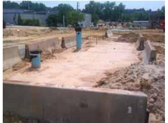
Fig. 27 Secured Ellipse Tank installation using Jersey Barriers.
