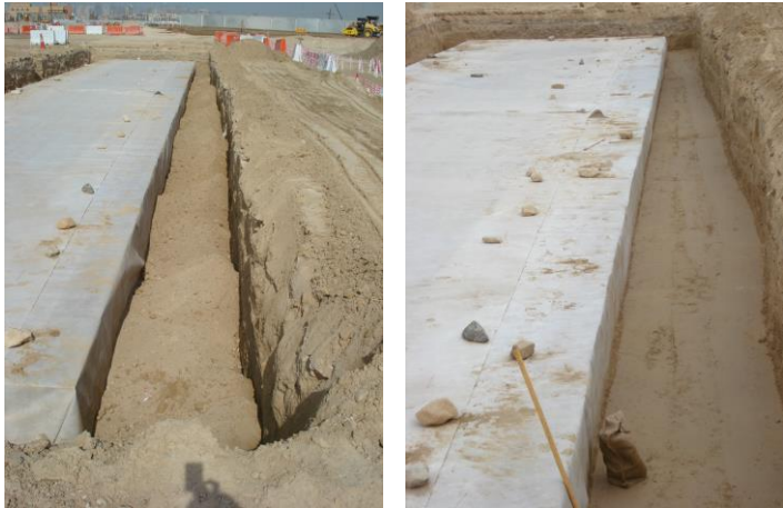
Fig. 23 Vibratory compaction of side backfill is always required , regardless of what backfill material is used.
