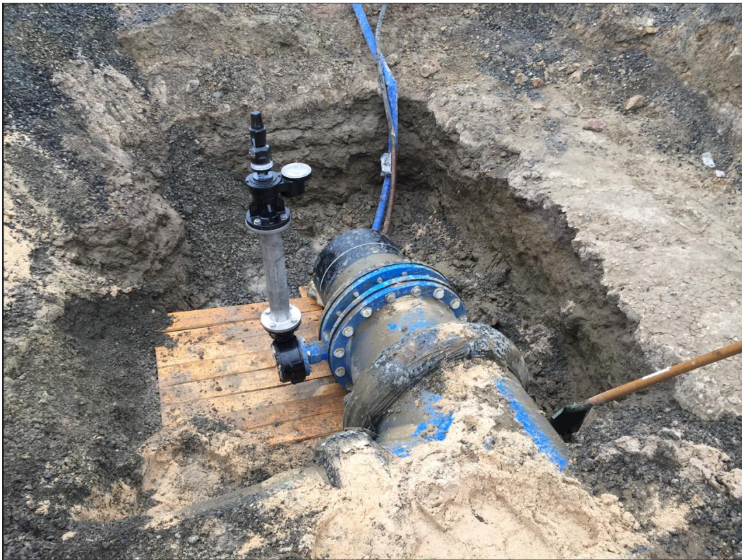
Figure 3: Challenger BFV buried installation with gear, torque limiter and dial position indicator
