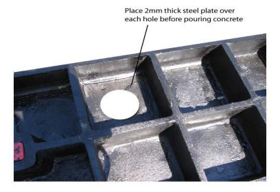
9. Fill rebates, cellular frames (Class D & G only) and recessed covers with concrete (minimum 32Mpa). Vibrate concrete and ensure all cavities and pockets are completely filled. The concrete must FULLY support the frame all the way to the inside edge. Trowel surface to achieve required finish.
